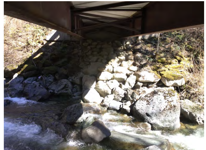
Left Bank Abutment when facing downstream
