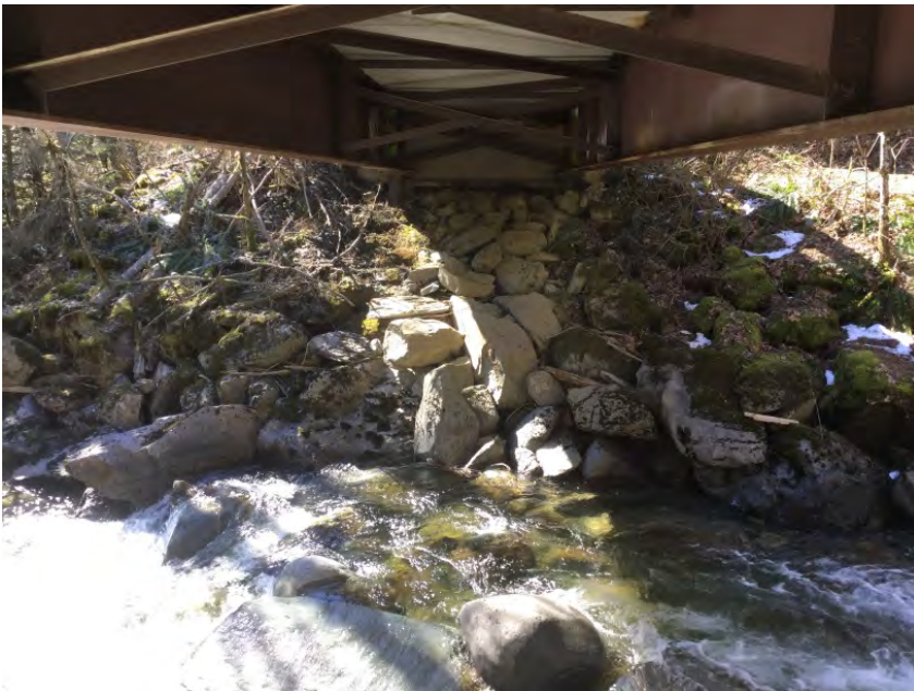
Right Bank Abutment when facing downstream
